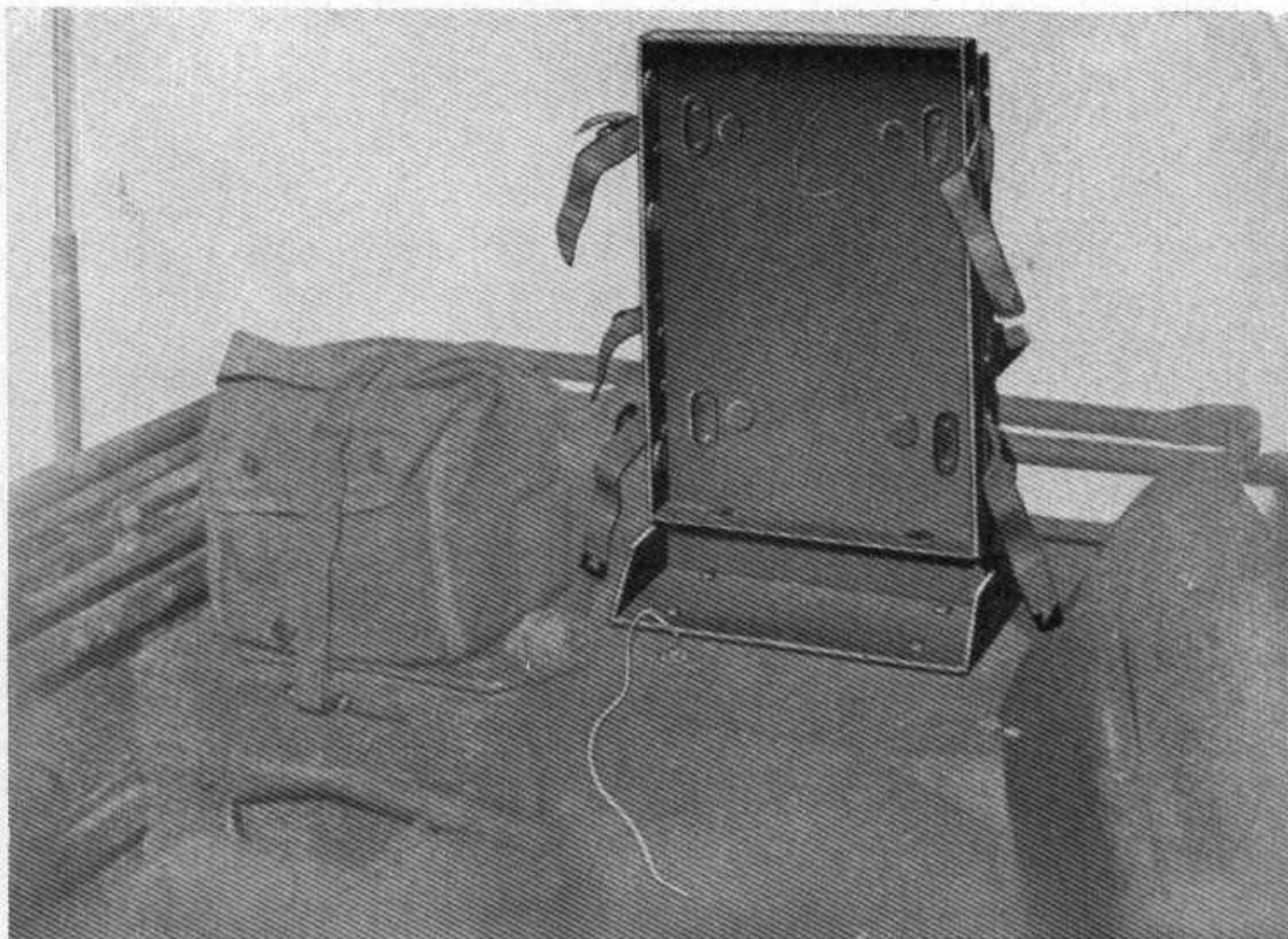
Figure 46. Mounting MT-350/GRC-9-GY and modified frame FM-85, installed in vehicle.
