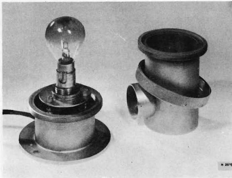
Fig. 59. Watertight light projector.
