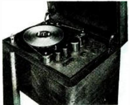
The recording or playback time of this magnetic recorder is 80 minutes. It employs a 1,000-yard-long plastic tape.
