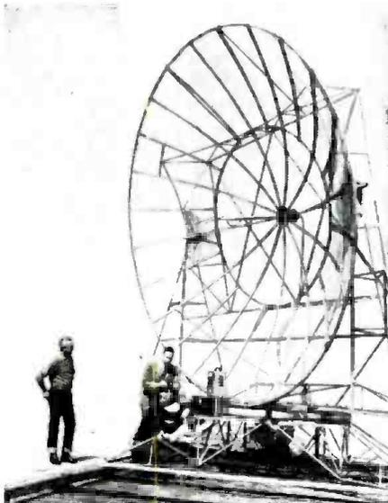
Used for reception of television signals from field pickup units, this parabolic receiving-antenna reflector is the largest in the U.S. It operates on a 100-foot track atop Mt. Lee in Hollywood, Calif. Constructed for the Don Lee Broadcasting System, the reflector stands 16 feet high. It can be pointed at any location in the surrounding area to pick up r.f.
