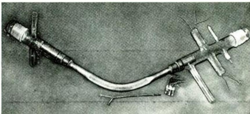
The analysis tube itself. The sample is injected into the transverse tube at the far right.
