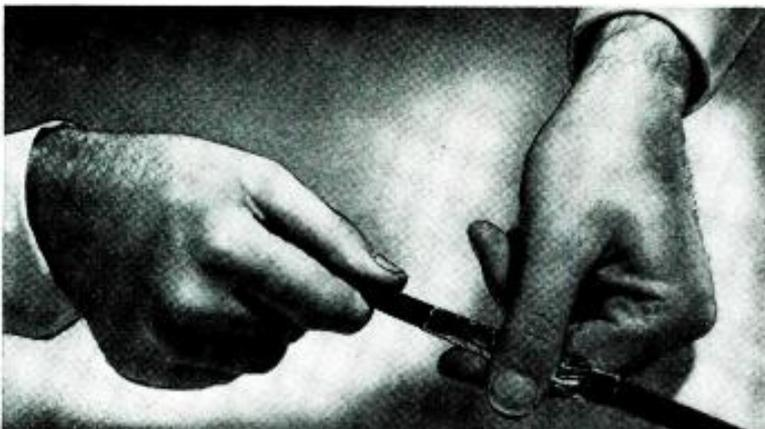
This photo shows the strip of tinfoil wrapped around the line and held in place with a clip.
