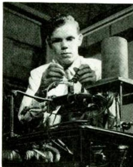
Loading sample chamber of mass spectrometer in preparation for an analysis of metal vapor.
