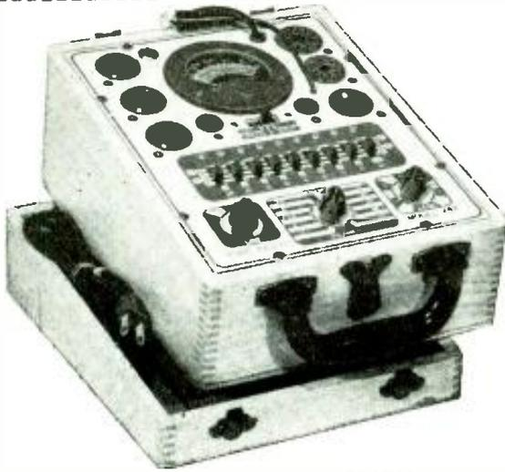
Model 247 comes complete with new speed-read chart. Comes housed in handsome, hand-rubbed oak cabinet sloped for bench use. A slip-on portable hinged cover is included for outside use. Size: 10 $\frac{3}{4}$ " x 8 $\frac{3}{4}$ " x 5 $\frac{3}{4}$ ".
