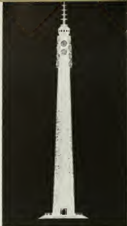
ANTENNAS TOPPING HIGH TOWERS SIMILAR TO THE ONE SHOWN HERE WILL RELAY TELEVISION AND OTHER SERVICES ACROSS THE COUNTRYSIDE.
