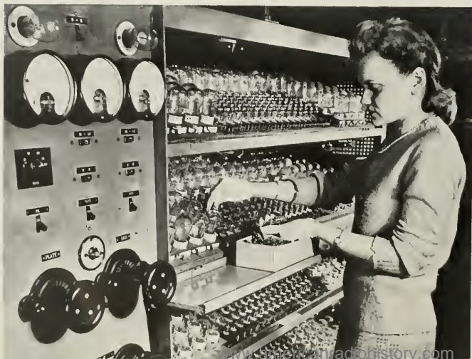
ABOVE: DEFT HANDS CEMENT CERAMIC INSULATION IN PLACE ON TUBE ELEMENTS. LEFT: SECTION OF THE AGEING RACK WHERE ALL TUBES UNDERGO SPECIAL TREATMENT BEFORE SHIPMENT.
