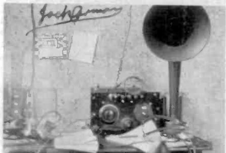
Figure 2. The receiving setup is similar to that shown in Figure 1, except that the left-hand tuning dial of the receiver has been changed from a vernier type to a direct-drive dial. This photograph is also dated "1929."
