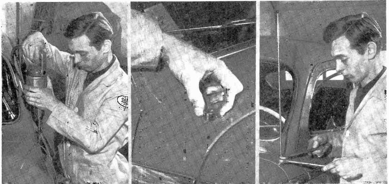
**Fig. 4 Steps in making a top cowl antenna installation. Left, hold the drill in vertical position to complete drilling operation; center, using mounting fitting as a template to determine location of mounting hole for a top cowl installation. This gives finished job custom fitted appearance. Right, tightening mast in desired alignment.**
