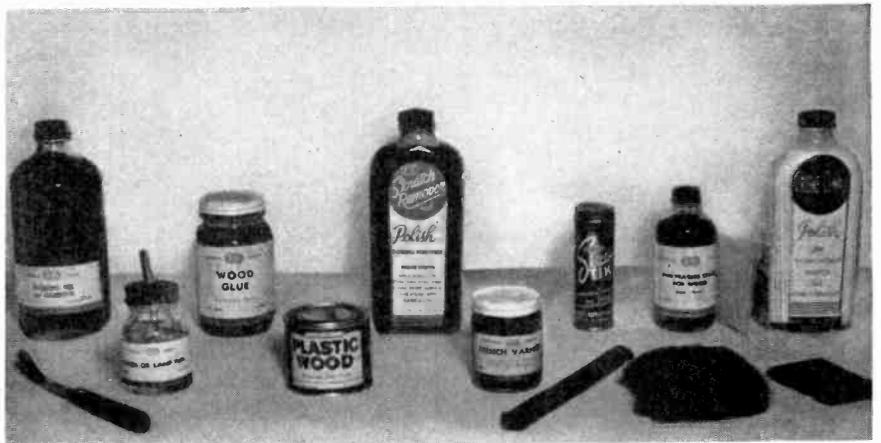
Fig. 1 These are the basic materials needed for cabinet repair work. From left to right they are: Rubbing Oil, Spatula, Alcohol Lamp, Wood Glue, Plastic Wood, Scratch Remover Polish, French Varnish, Stick Shellac, Scratch Stick, Stain, Steel Wool, Sandpaper, Polish, and a Felt Pad.
