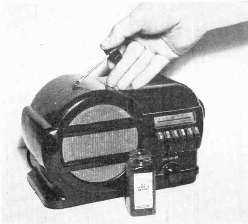
Fig. 9 Applying plastic cement to a gouged cabinet.
