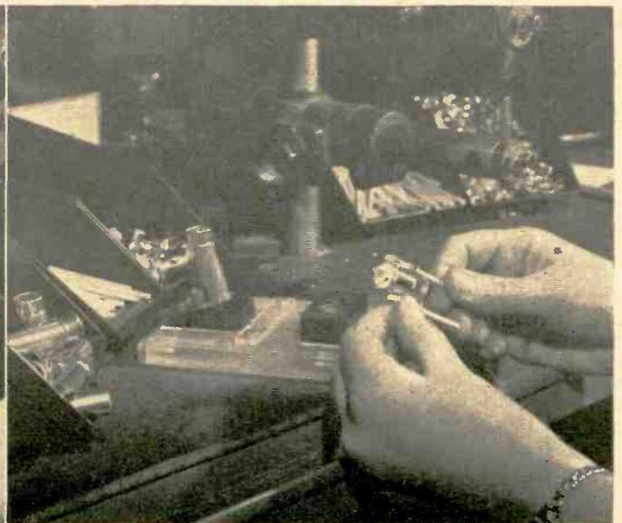
With all the inside parts in place, the CR tube, near completion, is evacuated and the exhaust tip sealed off in one operation (right.) Extremely high vacuum must be attained, in order not to impede the stream of high-velocity electrons. This process must result in vacuums much nearer to 100 percent than are needed in ordinary tubes.
