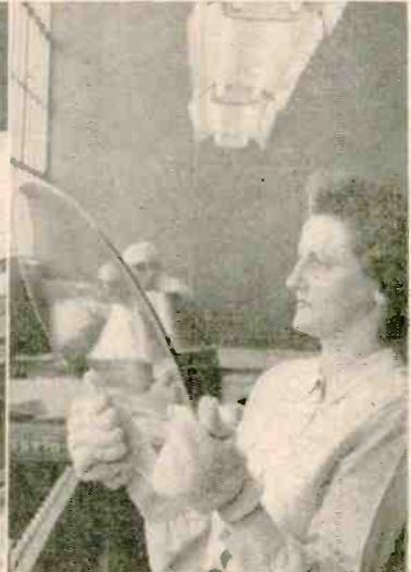
The new Du Mont 30-inch picture tube, shown at left, is not yet available in sets. It is said to be the largest picture tube made. Center: The last of 35 inspections made on every CR tube made in the plant checks characteristics and operation of the finished product, which is
