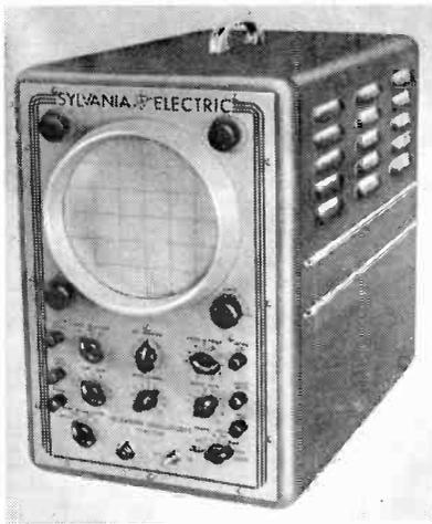
supplied with a 7JP1 green screen tube, provides a vertical sensitivity of ten millivolts per inch and a vertical response up to four megacycles.
