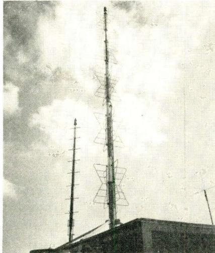
Antenna of Zenith's experimental Channel 2 TV station in Chicago, center. At left is the company's FM station antenna.
