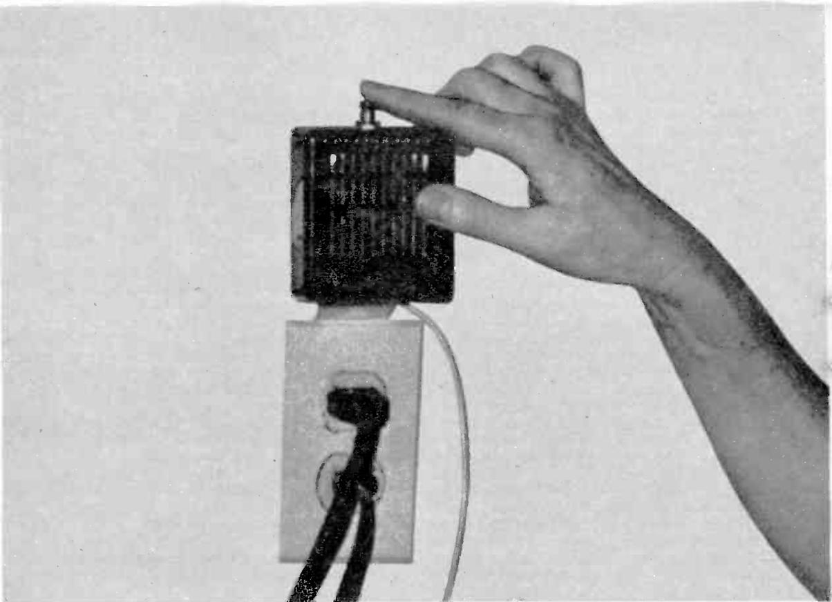
Tiny remote unit is attached to kitchen outlet plate, has convenient control switch on top edge. Indicated is one of three thumb-size transformers, in shot of partially-assembled master unit, left.
