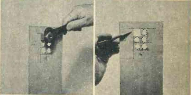
Shifted to second corner, punch trims off the opening right to the line. Overlap cuts if openings are not even multiples of punch size.
