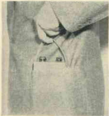
The transistor radio occupies only about half of an ordinary coat pocket. Its chassis fits in a small leather carrying case.
