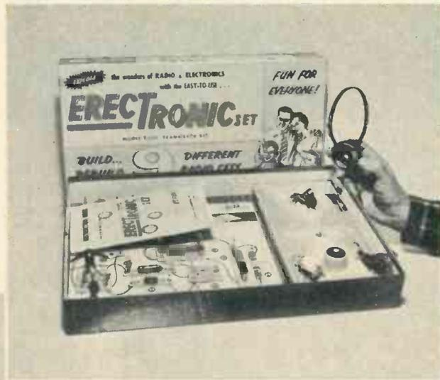
At left is a small tool-less radio kit, intended for persons entirely without previous knowledge of electronics. Some parts are already in position on the template over the baseboard. The larger kit, shown below, contains a tube, can be assembled into 15 different electronic units.
