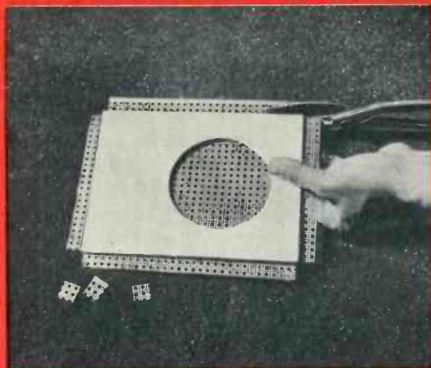
After cutting out speaker hole, cut Reynolds "Do-It-Yourself" Aluminum to cover plywood. Snip corners as shown.
