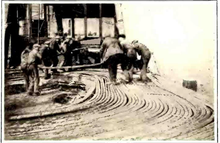
Uncoiling the sea-earth section of the new permalloy cable off Hammels Beach, near Rockaway. The cable weighs from 20 to 36 tons per mile and the men who handle it on the barge must show considerable dexterity to keep it from getting out of hand
