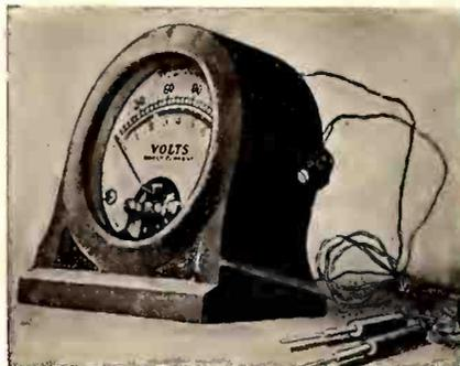
Shown above is a new Westinghouse high resistance DC voltmeter with a dual range, 0-7½ volts and 0-150 volts which will serve for measurement of either A, B or C voltages. Three foot leads are supplied with pin jack terminals for plugging in on any of the standard sets provided with voltmeter jacks
