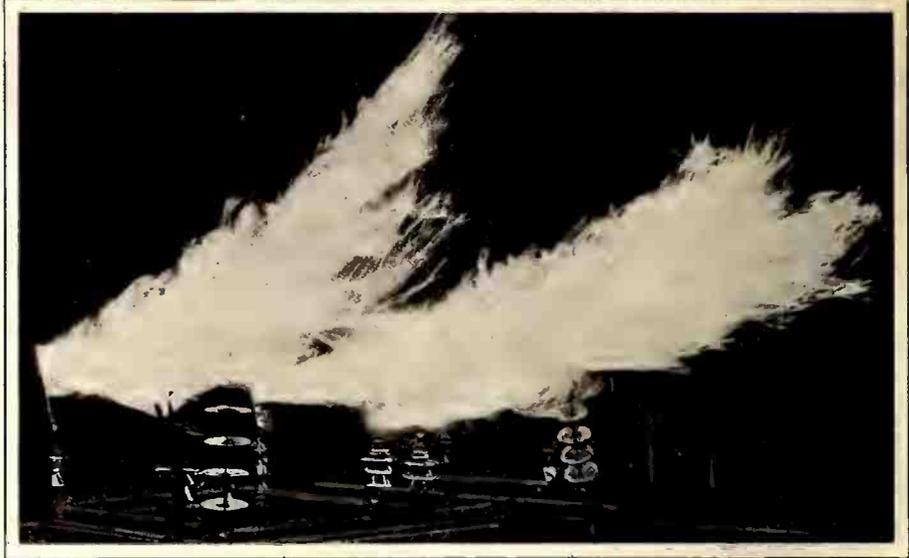
Above is shown the result of opening a disconnect switch on the modern 110,000 volt transmission line of the Georgia Railway & Power Company at Atlanta, Ga. This unusual view presents in graphic detail the tremendous power carried in present-day transmission lines.
