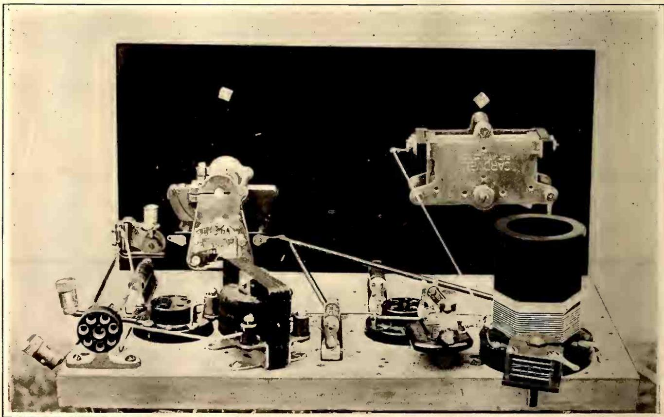
In this photo is shown the short wave receiver now used at 9BHX
