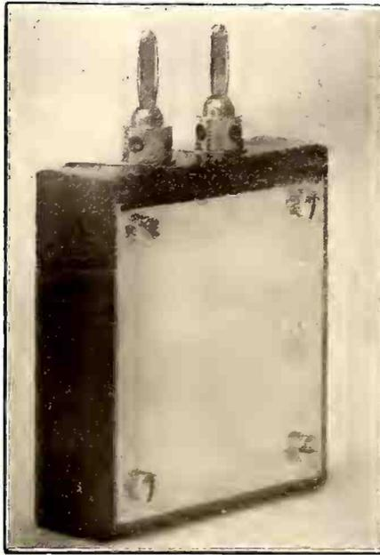
Quartz plate holder for piezo oscillator assembled
