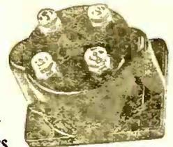
The famous S-M 210 and 211 Intermediate transformers, used in the receivers developed by McMurdo Silver and in several other well known designs, provide the highest amplification of any transformers on the market. Each transformer is laboratory-measured and supplied with individual curves—your guarantee of uniformity! The new bakelite case is especially attractive and efficient. Filter furnished with measured tuning condenser. Transformers supplied in sets of two 210's and one 211.
