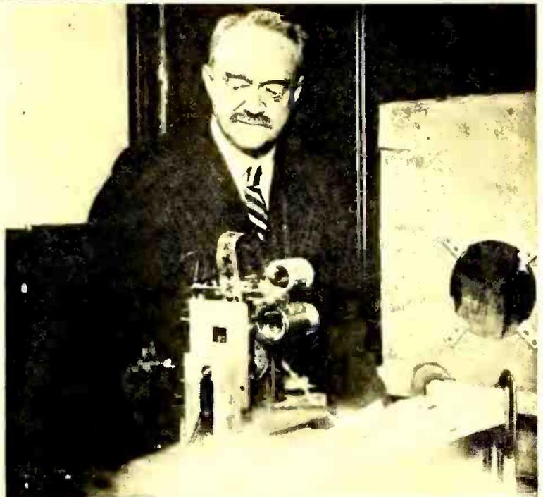
This photo shows Mr. Jenkins and the motion picture projecting machine carrying a scene of a Dutch windmill, the first movie object sent and received by radio.
