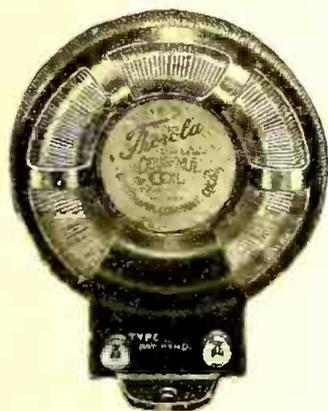
The new coil is of the toroid type, but differs greatly from all other coils of this type in that it shows extremely low losses. It was designed by Frank Reichmann, designer of the Thorola and Thorophone loud speakers, and marks the first step of the Reichmann Company into the general field of radio manufacture.
