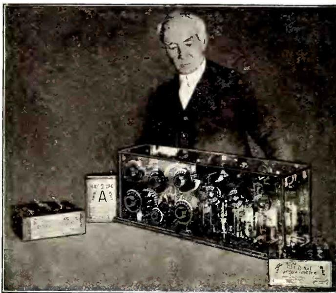
**T**HE French Battery and Carbon Company has the distinction of having in its employ Chief Designer John Graves, who has conceived and built a radio receiving set of glass with two steps of audio frequency. The set operates with 3 WD-11 tubes on a Number 1261B Ray-O-Vac "A" Battery and 3 No. 2151 Ray-O-Vac "B" Batteries on the plate circuit.
