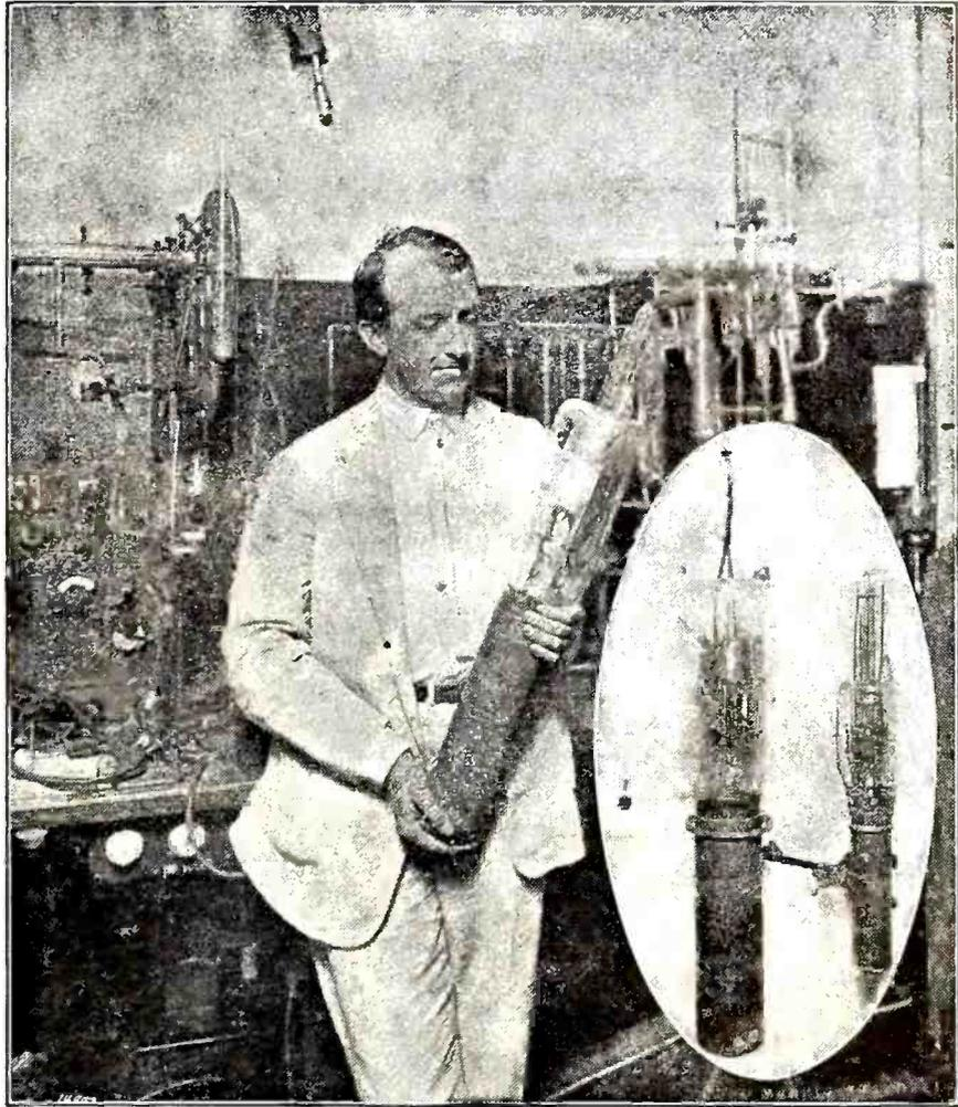
*W. G. Housekeeper, the Western Electric engineer whose epoch making invention led to the production of the world's largest vacuum tube, and the tube itself. Insert shows in graphic fashion just how the new monster tube compares with the little "peanut" tube used in the average radio receiving set and the 10,000 watt tube which only recently was considered the last step in this department of science.*
