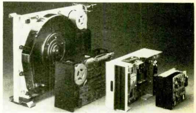
The complete line of Shugart Associates' fixed and floppy disk drives, from the big 14-inch SA4000 down to the SA400 Mini-floppy. The two drives in between are both 8-inch.
