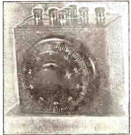
The Benson Melody Wave Trap eliminates annoying interferences. It is the inductively coupled type with a high grade .001 mfd. variable condenser. All mounted in a beautiful leather covered cabinet with an engraved bakelite panel.
