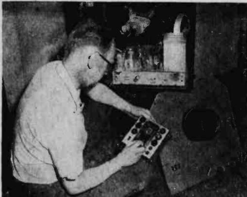
The professional service technician usually checks tubes by substituting new tubes for those he knows from experience to require most frequent replacement. He also tests certain tubes for grid emission with the grid circuit tester. Grid emission is a very frequent cause of TV ailments and is not readily detected with general-purpose tube testers.
