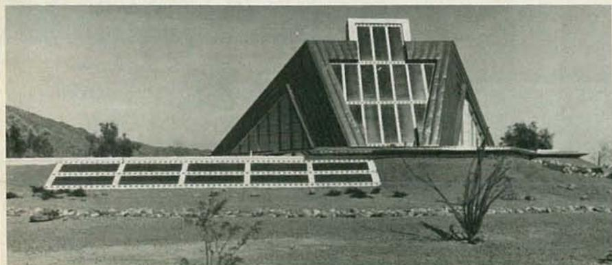
DESIGNED TO FIT its mountain and desert surroundings, the *House of Dreams'* unique features include solar collectors for heat and hot water supply and high earth banking against both heat and cold. (The Ahwatukee House has other non-electronic unique features. For example, there is not a square room in the house.)
