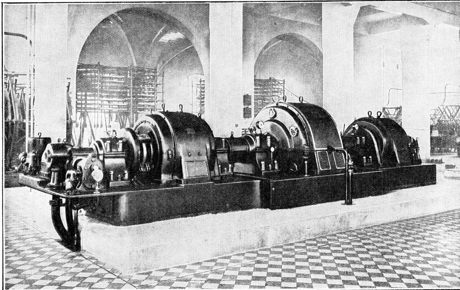
ALTERNATEUR FRANÇAIS A HAUTE FRÉQUENCE DE 500 KILOWATTS, INSTALLÉ AU CENTRE D'ÉMISSION DE SAINTE-ASSISE (SEINE-ET-MARNE)
