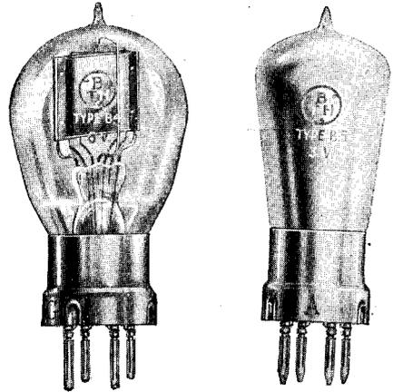
Types "B.4" and "B.5" dull-emitter valves manufactured by British Thomson-Houston Co. Ltd.
