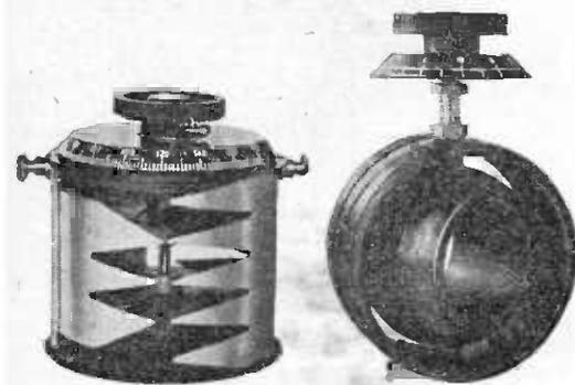
*Maxone variable condenser with specially shaped plates and variometer by Messrs. J. Macdonald & Co.*
