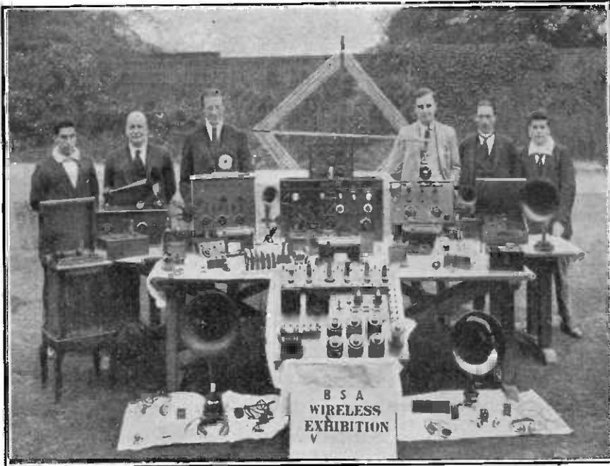
*The display at the Club's first exhibition on September 1st. All the apparatus shown was constructed by the members, with the exception of the Burndept "Ethophone V" on the left, and the two-valve panel in the top centre.*
