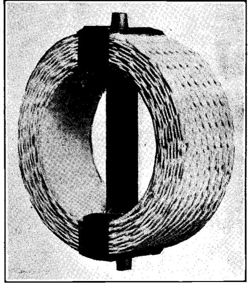
Fig. 8. This is probably the best method of joining the ends of a coil.
