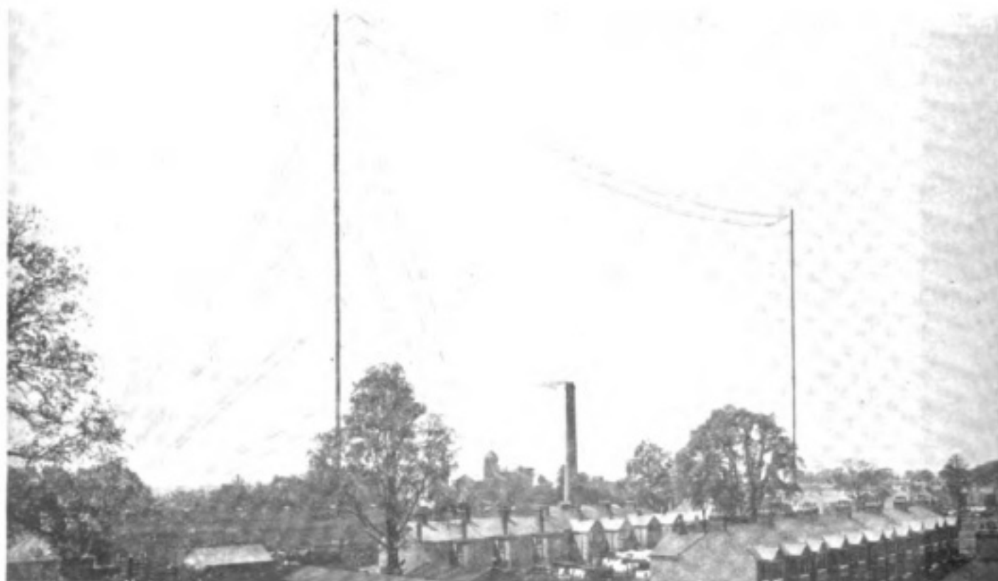
The Masts (475 feet high) and Aerial at the Marconi Works, Chelmsford, which are used for the Wireless Telephony Demonstrations.
