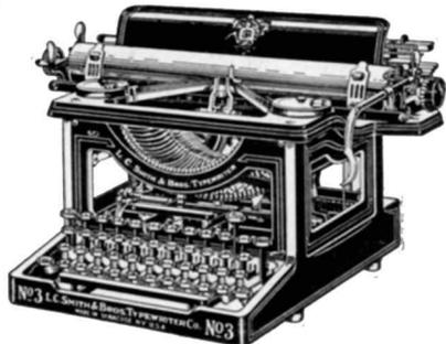
L. C. Smith & Bros. Typewriter has Ball bearings, serving exactly the same purpose as the Jewel bearings of an expensive watch. Ball bearings, not only for the Typebars, but at all important wearing points; of course this reduces friction, noise, and wear, and makes the machine easier to operate.
