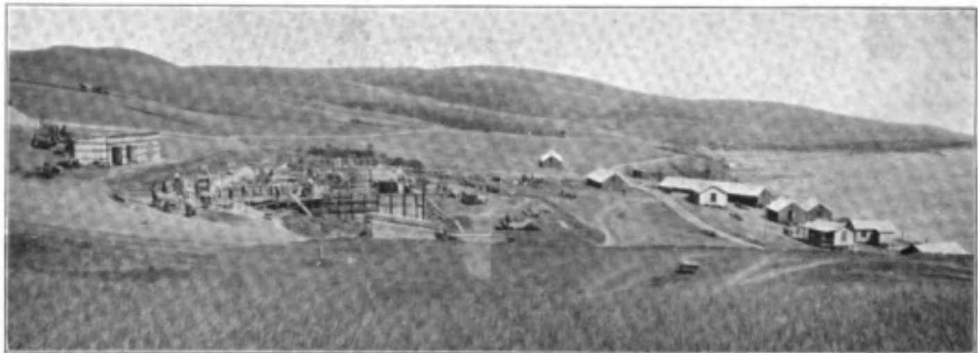
San Francisco Transmitting Station.
