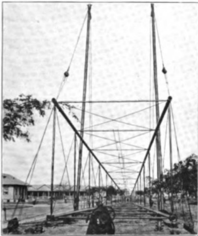
The first mast of the Trinidad Wireless Station ready for hoisting.
