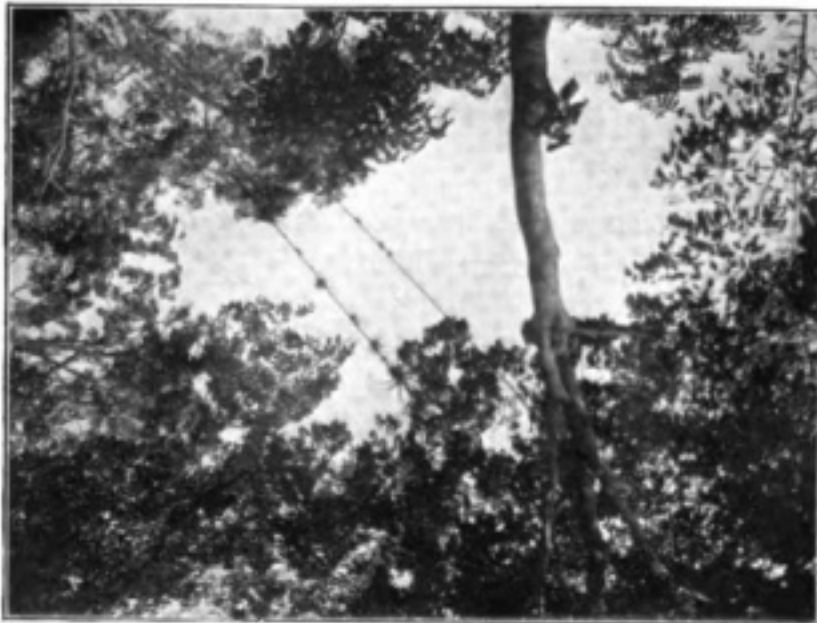
Luxuriant vegetation destroying a cable.
