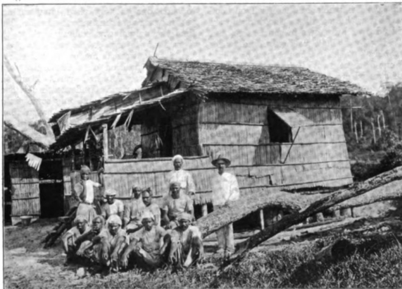
Mr. F. Post, and his gang of Lascar labourers engaged in Mast Erection.
