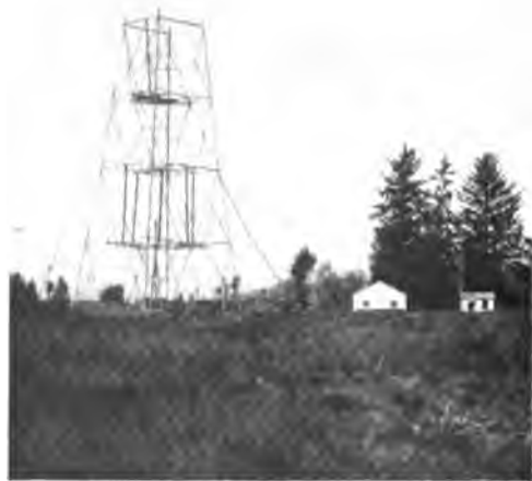
Astoria Station—Two forward Towers under construction.
