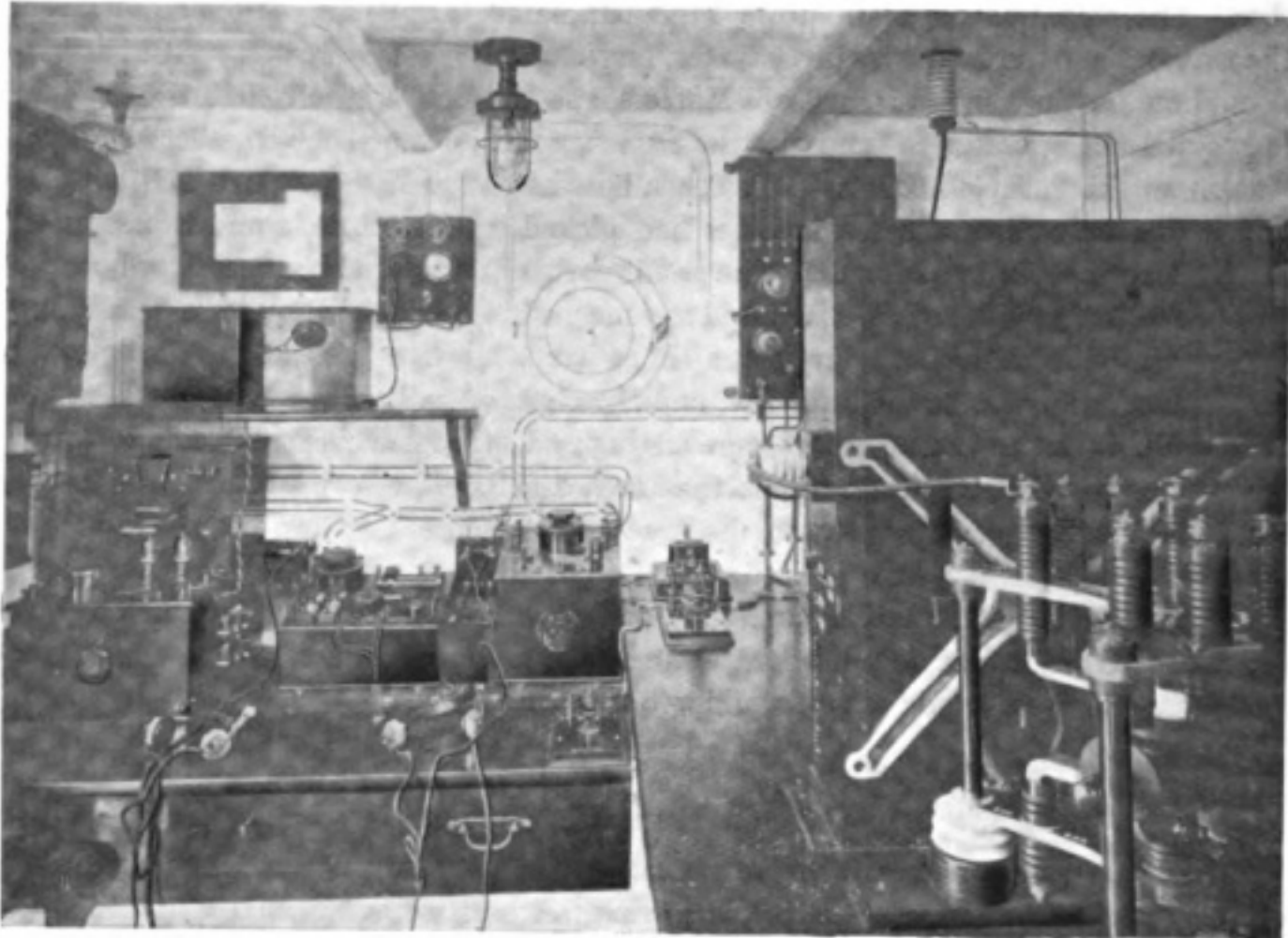
RECEIVING APPARATUS ON BOARD THE SPANISH GUNBOAT " BONIFAZ."
