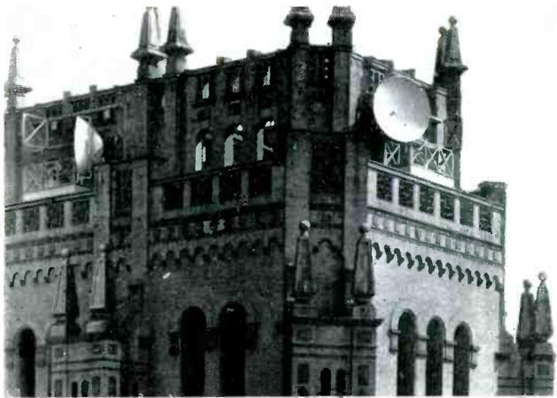
Fig. 1. Antennas and reflectors for micro-wave signals used in P.T-M system resemble searchlights as seen in this photograph of the mounting of two such antennas at the top of the International Telephone Building in New York City.
