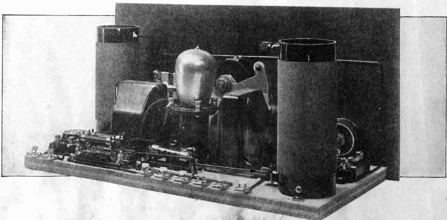
moving one of the small bolts securing the stator plates of the variable N condenser and fastening the fixed condenser to the N condenser by means of the bolt.
