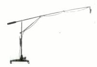
two telescoping four-foot sections, the boom (RCA Type KS-4A) has a controlable arc of approximately 180 degrees, and is counterbalanced so that it may be freely elevated and rotated to any point within its range. The sturdy stand is of all-steel construction with satin chrome finish, except for the low gravity cast iron base, which is finished in dark umber gray.
