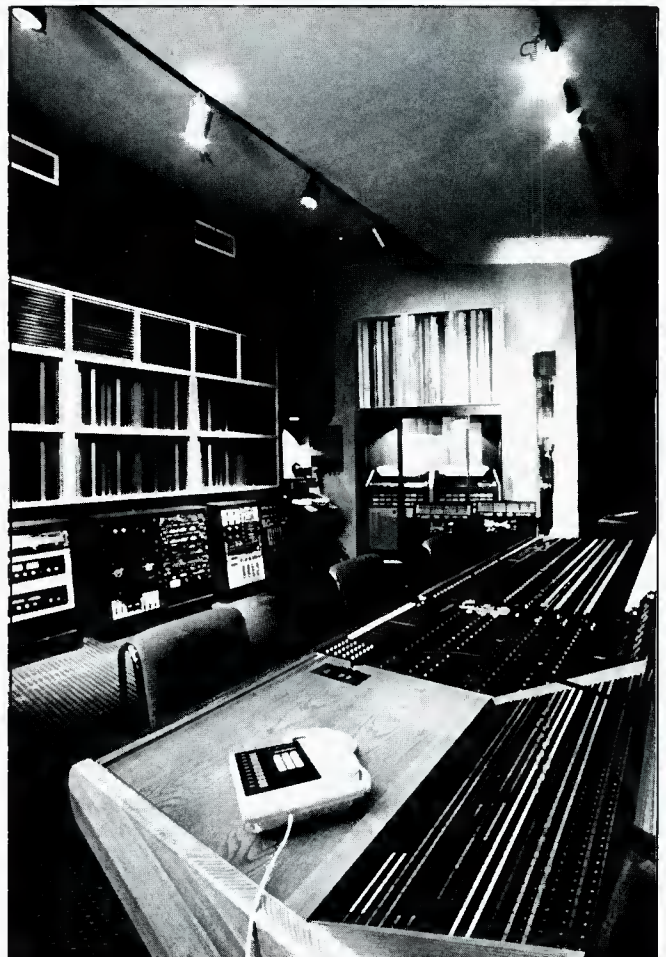
Figure 5B. Rear view of the control room at Master Sound Astoria in the Kaufman Astoria Film Studios, Astoria, NY, showing rear and side RPG diffusors. Acoustical consultant, Charles Bilello Associates.
