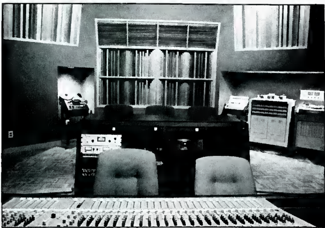
Figure 5D. RPG rear wall at Welk Music Group, Nashville, TN. Acoustical consultant Bob Todrank, Valley Audio. A special corner LFD, shown in Figure 8 is positioned behind the central RPG cluster.
