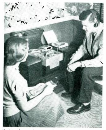
No internal connections are made on the recorder. Monitoring can be done on some machines with headphones, as can late-atnight listening.
