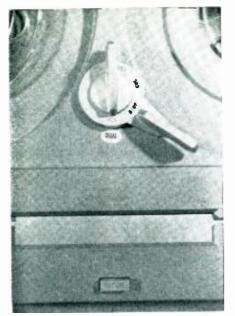
All mechanical controls are centered in this one unit. The smaller lever controls the fast forward and rewind; the larger the functions such as run, cue, edit and stop. The record safety button can be seen below tape gate.
