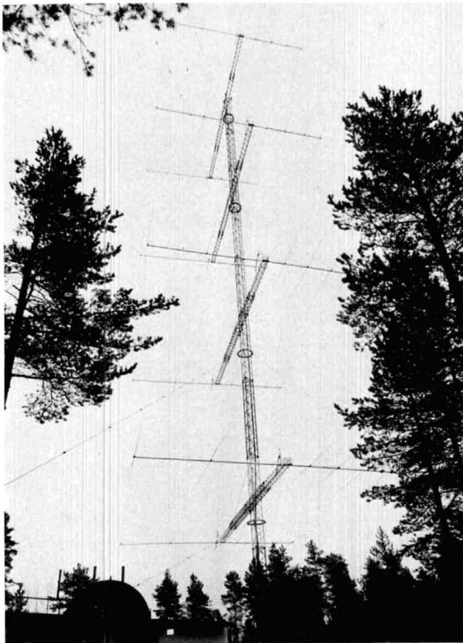
**fig. 5. The monster 20-meter array of Simon, OH8OS. The antenna consists of eight six-element beams, stacked two-over-two. Simon puts through an S-9+ signal on the West Coast of the USA when other Europeans are inaudible. The complete tower is rotatable.**
