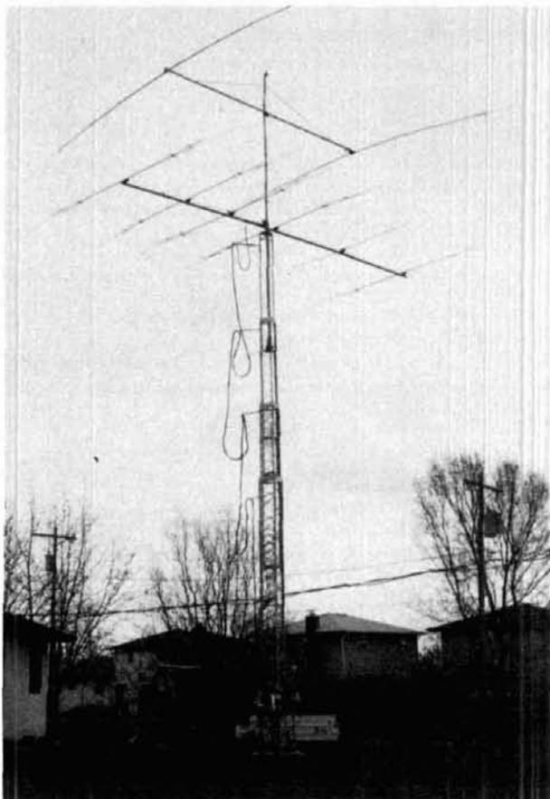
Set in 7½ cubic yards of concrete, author's 70-foot Tri-ex 470D tower is completely self-supporting, with fully motorized crank-up, tilt-over capability. Lower antenna is a KLM KT34XA; upper antenna, at 80 feet, is a two-element Cushcraft 40-meter beam. Both were erected by K8RA without assistance.
