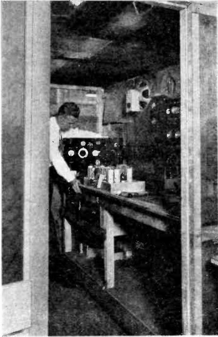
*Left, Fig. 6: One of the shielded cages on the set floor of the Pilot plant, where assembled chassis are tested thoroughly with equipment of the very latest design and construction. The apparatus in each of these booths costs more than a thousand dollars.*
