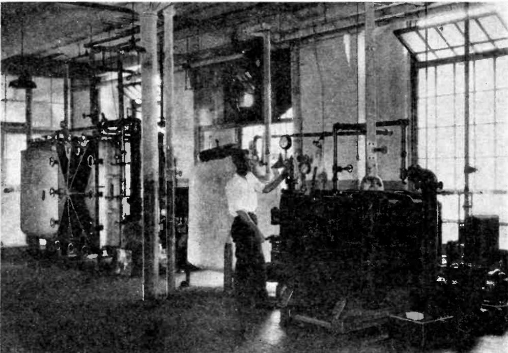
Fig. 1: A section of the condenser department, showing the large storage and impregnating tanks used in the manufacture of fixed condensers of various kinds.
