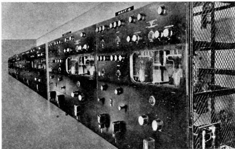
*This is what the voice-and-television transmitters of stations W1XAV-W1XAU, of the Short-Wave and Television Corp., Boston, Mass., will look like when they are finished. W1XAV, on 2,870 kc. and 1,000 watts, is transmitting 60-line, 20-image television. W1XAU, on 1604 kc. and 500 watts, broadcasts voice simultaneously with the images. Two other units will be devoted to relay broadcasting on 6,040, 11,800, 15,250 and 21,460 kc.*
