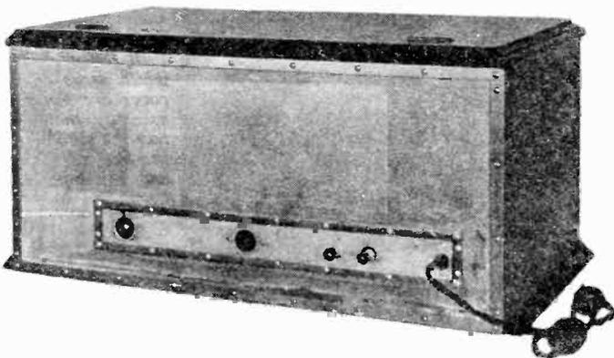
*Back view of the "All-Wave" receiver purchased by the King of Siam. This is a stock instrument except for the special nickel-plate mesh back.*
