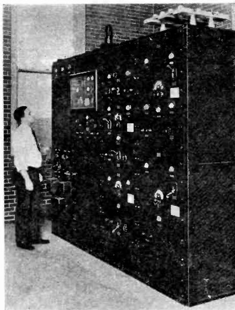
*This illustration shows a section of the equipment recently installed in the new Westinghouse transmitting station of KDKA located near Saxonburg, Pennsylvania. This apparatus is for use with the short-wave transmitters. Shown in the photograph is the crystal control equipment, as well as the frequency multiplying and amplifying apparatus. This panel is of the very latest design and will insure accurate maintenance of frequency.*
