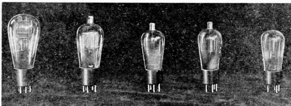
Left to right: the 247 power pentode, the 551 variable-mu, the 237 screen-grid, the 238 power pentode, and the 236 general purpose tube.
