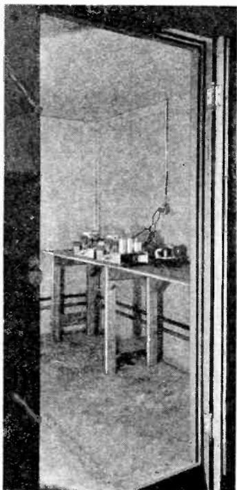
*Looking through the door of the "Torture Chamber" into the iron-lined inside. Two receiver chassis are on the table undergoing a heat and humidity test.*
