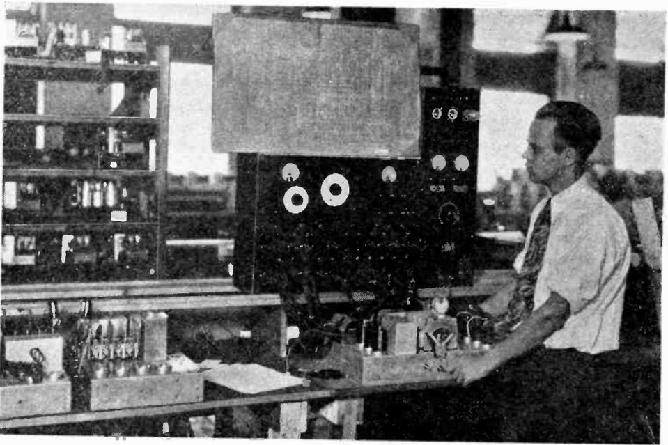
*Above, Fig. 4: The ingenious continuity testing board, which indicates the condition of every circuit in a receiver. After a set comes off the assembly line it is passed on to this board before it goes to the shielded test booths. Minor errors in wiring or adjustment are quickly detected, and the necessary repairs made without delay.*
