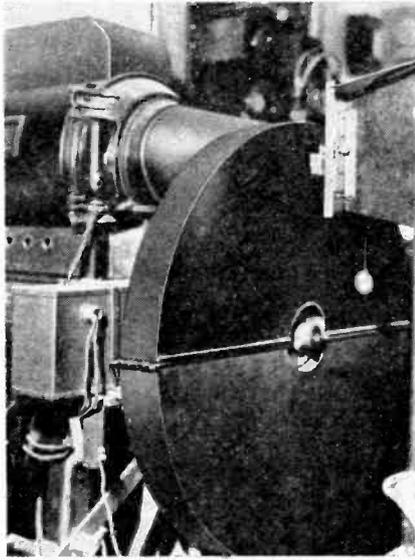
*Above: A close-up of the enclosed scanning disc used in the W2XBS television transmitter. Behind it is the arc light, and in front the opening in the frame that holds the photoelectric cells.*
