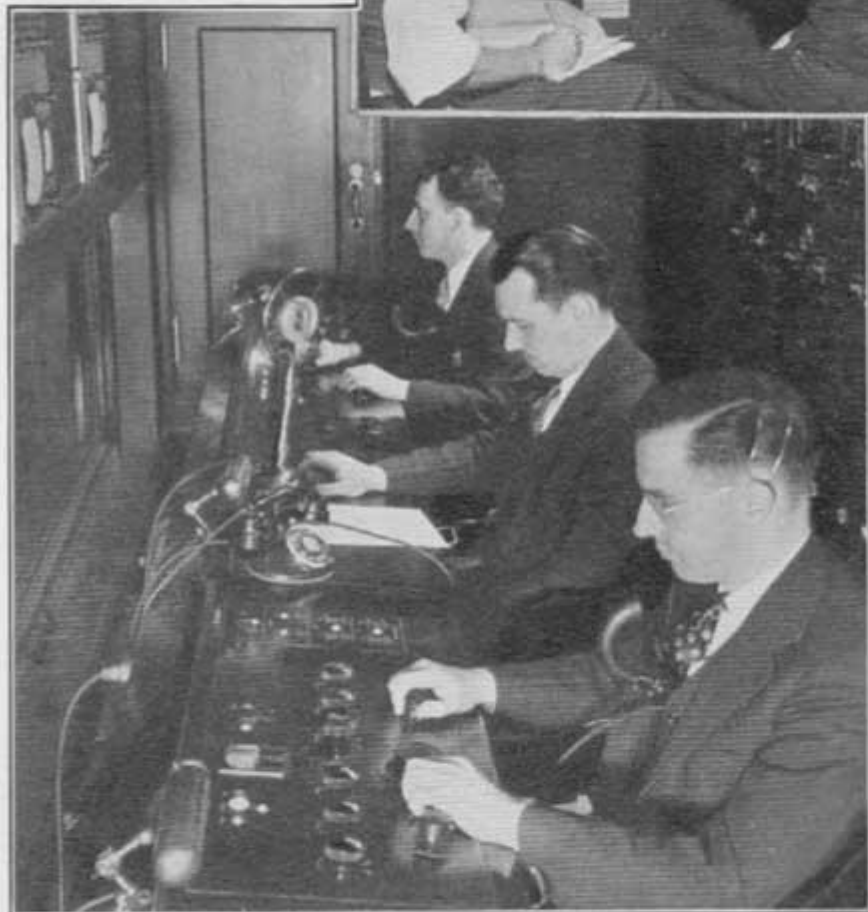
FIG. 3. CONTROL ROOM, NBC STUDIOS. ENGINEER IN FOREGROUND MONITORS SOUND FROM STUDIO MICROPHONES; AT FAR END IS THE VIDEO MONITOR; CENTER, PROGRAM DIRECTOR, FACING TALK-BACK MIKE, INSTRUCTS TELEVISION CAMERA MEN, WEARING HEADPHONES, IN STUDIO.
