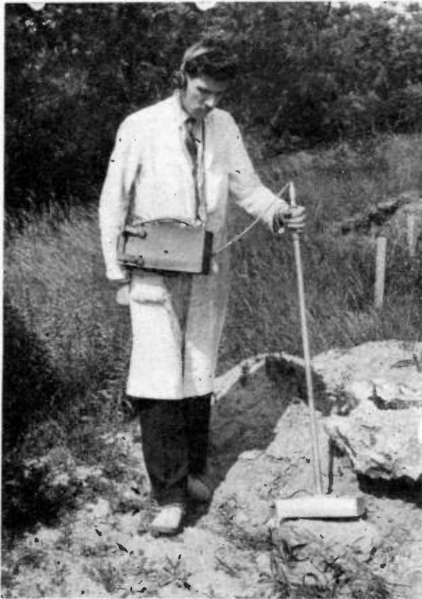
FIG. 2 b. — GAMMAMÈTRE POUR PROSPECTION AVANCÉE AVEC SON BLOC DÉTECTEUR.
