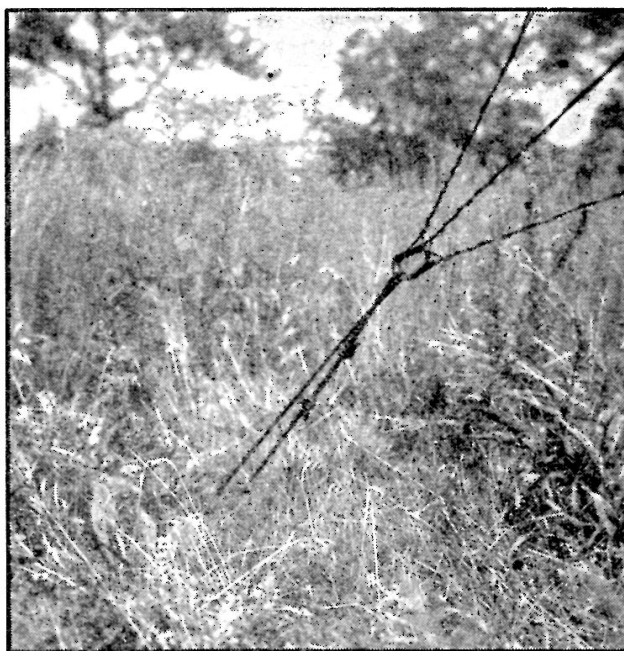
Fig. 1614 — An open thimble provides a method for hooking several guys to a "dead man" anchorage, and avoids sharp bends in the guys at the junction. This installation is at W2DC
