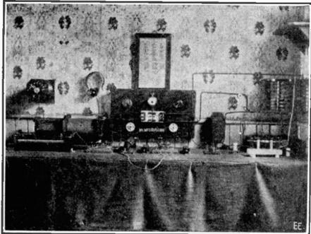
My receiving set consists of tuning transformer, double slide tuning coil and a loading coil, with galena detectors, variable and fixed condensers and 1,000 ohm Murdock phones. The aerial has four wires, 60 feet long, suspended on two poles; one 40 feet high and the other 32 feet. My ground is of iron buried in the earth. I am quite satisfied with
