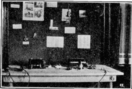
The detector is to the right of the variable condenser which is of silicon type and a fixed condenser is used also. I also have a buzzer test.
