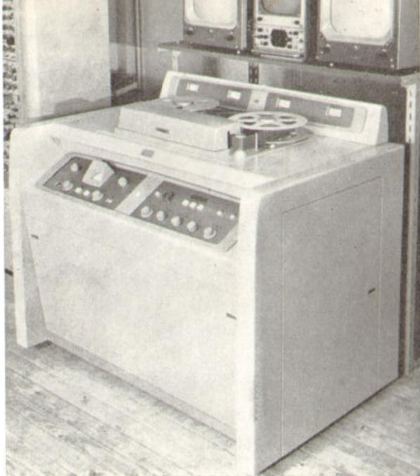
Le Videotape Recorder Ampex VR 1000 (photo C.F.T.H.)
