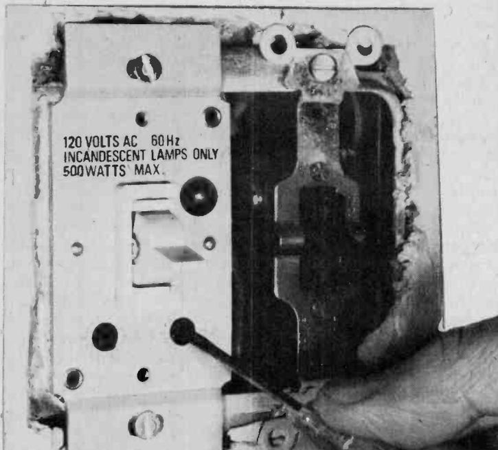
There's even a replacement module for wall-switched lights. You can still operate your lights independently of the X-10 with this switch. Circle 70 on the reader service coupon for more info.
